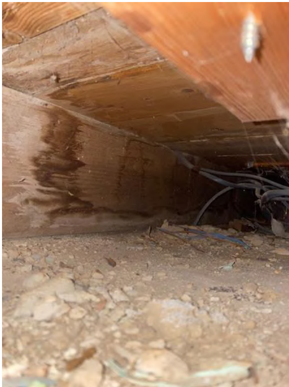
Sub floor wet room (photo provided by tenant)
