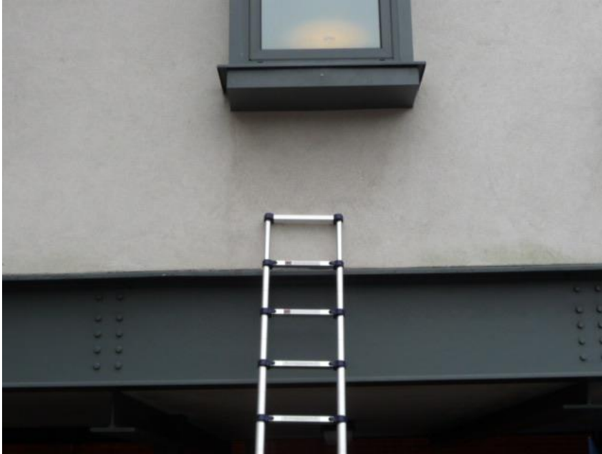
24 This home on a flood plain was built on steel uninsulated stilts in direct contact with uninsulated floor
