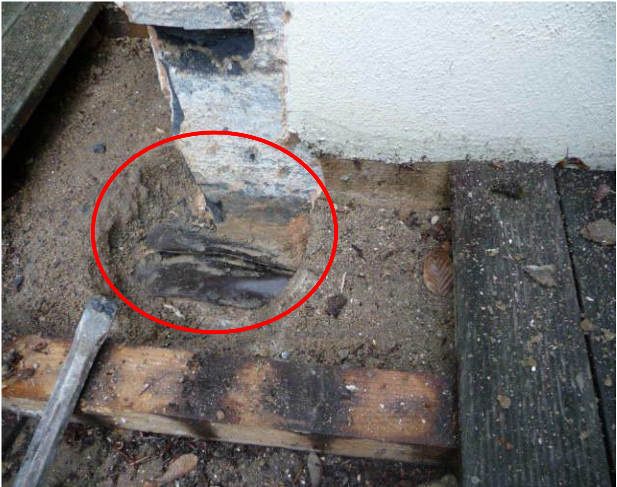
33 The damp proof membrane (DPM) did not rise high enough and the walls were saturated from penetrating and rising damp
