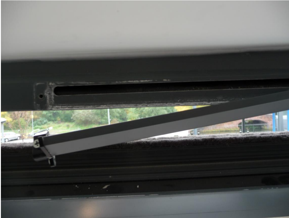
30 Despite having tickle vents visible they were not installed properly as they did not penetrate the window
