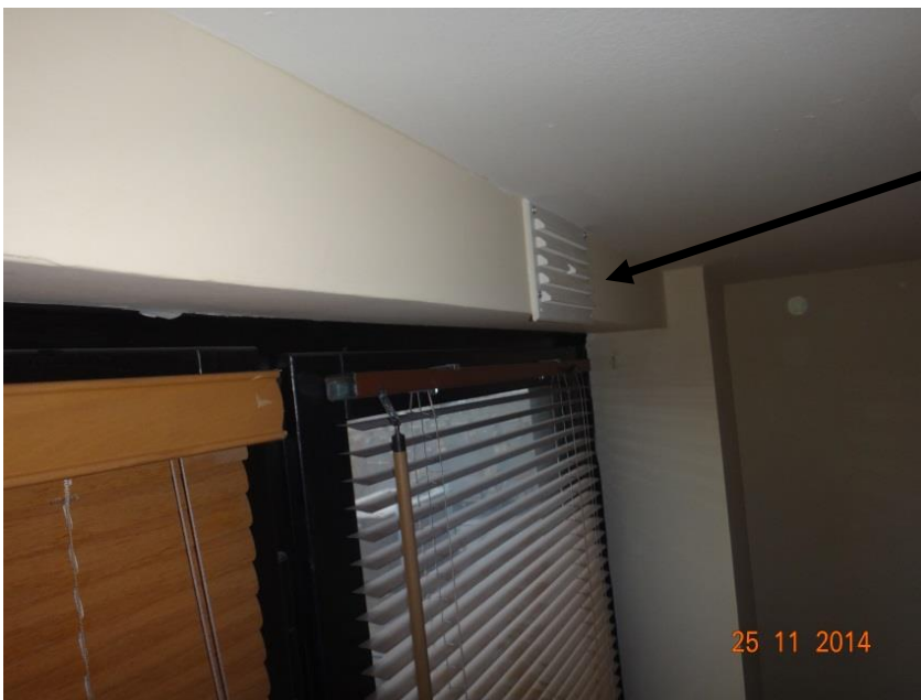
30 The kitchen vent didn't appear to control ventilation (see photo 31)
