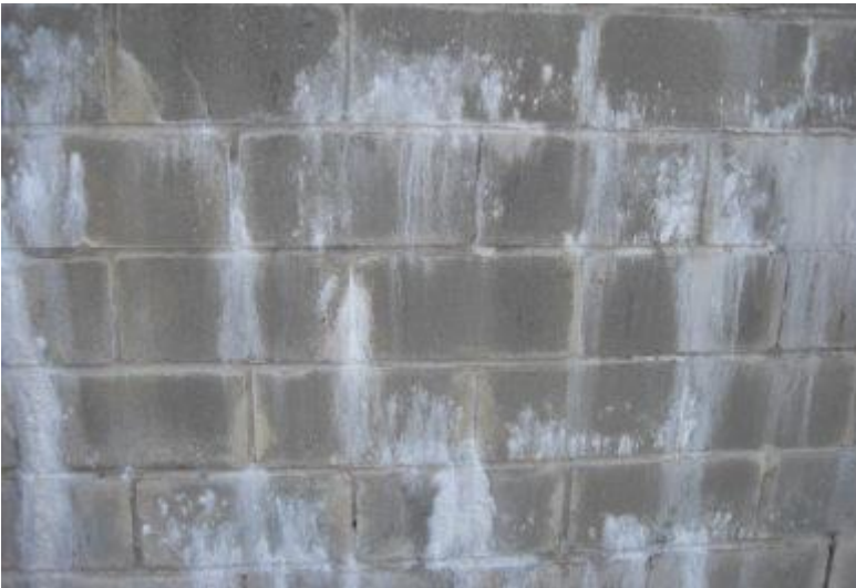
18 Chloride and nitrate salts of sodium give false wet readings
