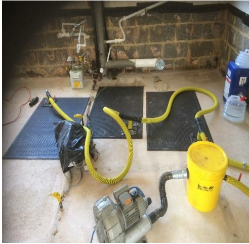
Using vacuum systems to dry and decontaminate
